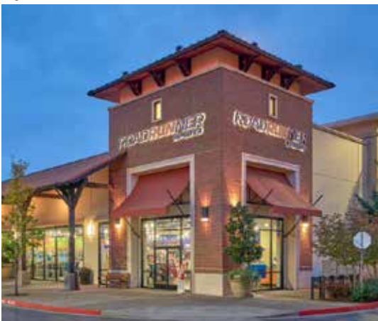
Clear delineation of building entries
