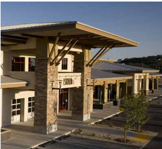
Projecting architectural elements
