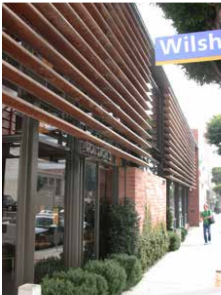
Clear walkways along building facade
