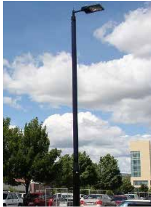
Parking Lot Lighting
